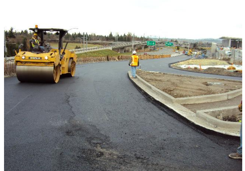
CRCF ORI 518 On Ramp Paving
