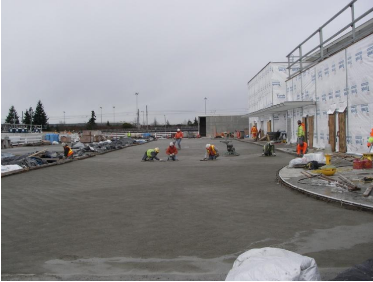
Bus Drive Lane Topping Slab Placement
