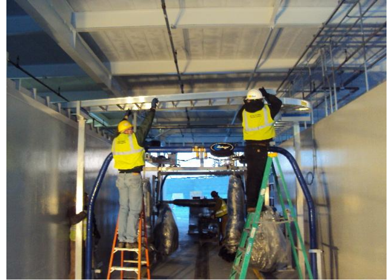
QTA #1 Car Wash Equipment Installation
