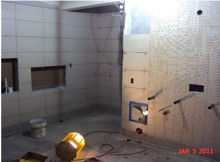
CSB Restroom Tile Placement
